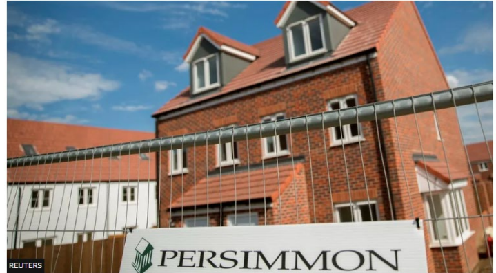
The UK's second biggest housing firm does not have an agreed minimum standard for all the homes it builds, an independent report has found.
